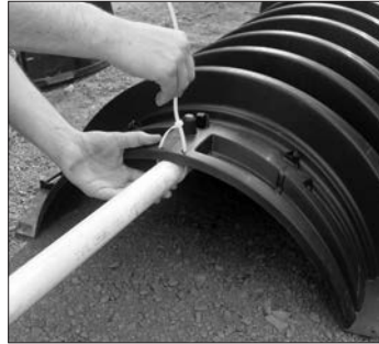
5. Secure the pressure lateral pipe.
