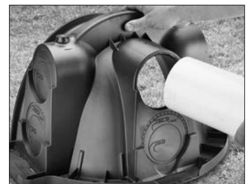
5. Insert inlet pipe.
